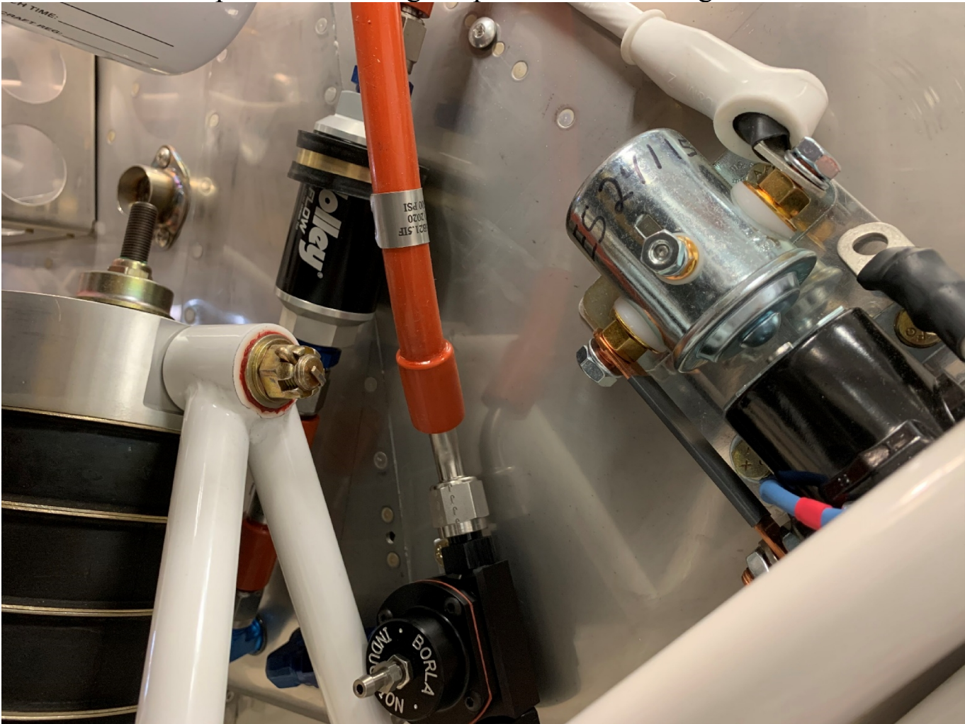
Another Firewall picture including the post filter mounting location.
